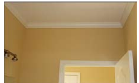
Crown molding runs throughout the home.
