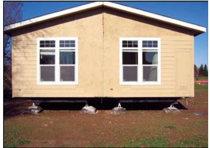
The double section HUD home is set on a Sure Safe EFS foundation for compliance with the new Federal Fannie Mae and FHA guidelines.
