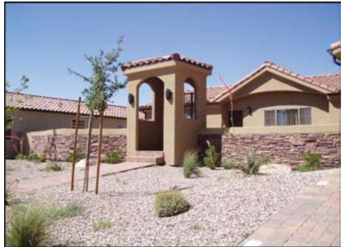
Completed homes finished with FHA approved permanent foundations by Sure Safe EFS and carrying FHA insured mortgages with 3.5% down-payment. HUD-Code homes were sold and set by Jeff Erickson of Quality Wholesale Homes, St. George, UT.
